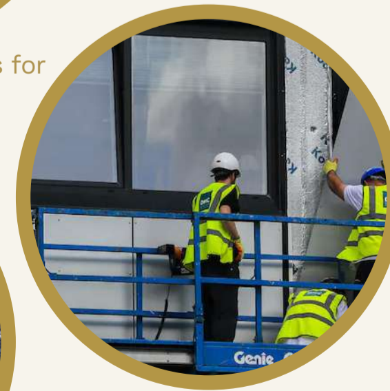
Upgrades to thermal wall insulation
