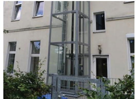
Example of external lift addition from HTA Design Berlin Study Trip, September 2015.
