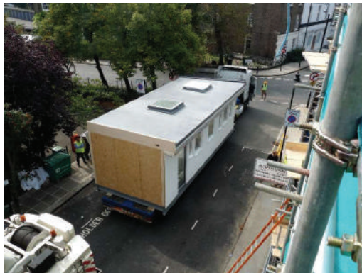
Delivery of pre-fabricated pod construction to Wilmot Place by Apex Airspace Development Ltd
